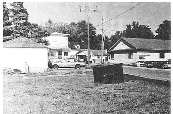
View from Ann Street to Main Street. Note the new alignment would greatly improve the skewed intersection at Main Street.
