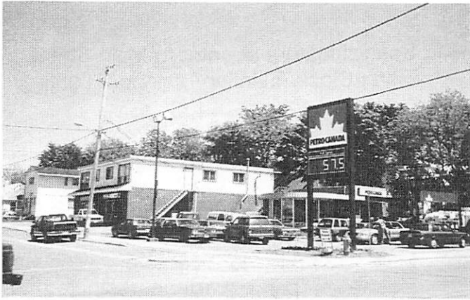
View of existing station
